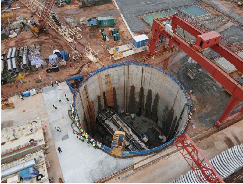
Figure 2: Northern portal TBM (TBM 01) sinking shaft
