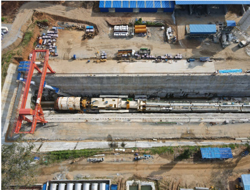
Figure 3: Southern portal TBM (TBM 02) ready to excavate
